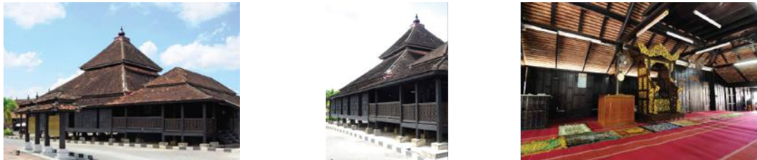
Figure 2. Images of Kampung Laut Mosque, Kelantan (Al Fozan Mosquepedia)
